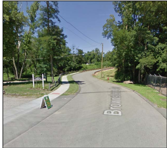
Brownstone Avenue Connection (looking northeast)
