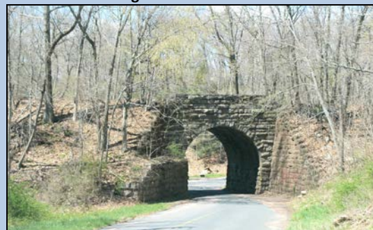
Railroad Bridge Over Middle Haddam Road
