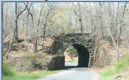
Railroad Bridge Over Middle Haddam Road
